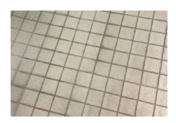
The required work consists of acid washing of both shower areas to etch and/or remove any remaining grout and re-grouting. To minimize the time the pool area is closed, proposals were solicited with only Hadi Construction Co. quoting, in the amount of \$8,600.
