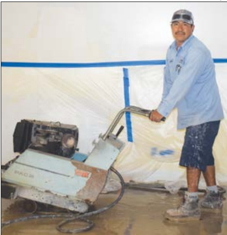
Jaime Morales of Service Maintenance is using a concrete grinder to prep flooring as part of the complete overhaul of a room in Clubhouse 3 that will soon be the site of a demonstration kitchen. It will be used in cooking classes as part of the new Learning Center that is coming to Leisure World.
