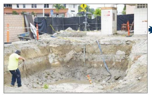
Work is now underway on the pool and spa reconstruction project. Starting June 25, crews, working under the direction of a soils engineer, drained and filled the hole left by the old pool, laid fabric cloth (lower left) and gravel before compacting the site (lower right). The pool will be relocated to make the most of the site. The facility will include a pool with five swimming lanes, an activity area and a spa, among other features.
