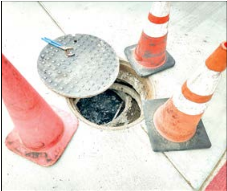
A blocked Mutual 9 sewer line is undergoing repair.
