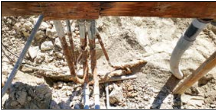
A corroded conduit to the Leisure World Golf Course lake pump and men's and lady's pool locker rooms has been replaced.
