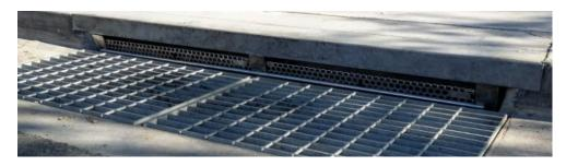
\* Leisure World's curb opening heights are shorter than typical. ARS-CL screens that hinge and swing inward may not be the best option. FXSS customized fixed screens are made of the same ARS-CL materials but have no moving parts. There is no concern of flooding due to fixed screens since all locations have grates in front.
