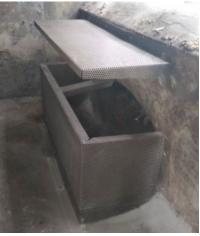
A. **G2 CPS-Mod™** patented **Connector Pipe Screen** *Full Capture System.* 304 Stainless Steel with 5mm filtration holes. Installed inside the Inlet catch basin around the discharge pipe.
