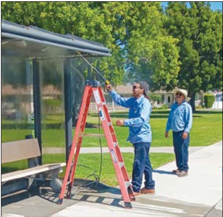
Service Maintenance team members Alex Acedo (l) and Juan Fuentes (r) remove peeling paint and rust from a LW bus stop in late July.
