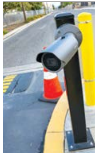
Each gate is equipped with license plate readers.
